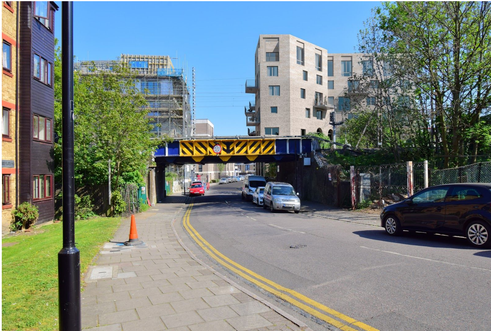
View from the West side of the railway bridge (Leaside Road)
