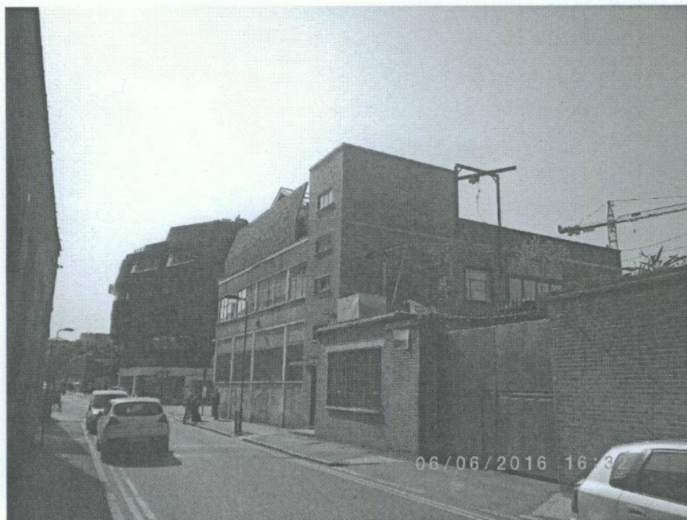
East elevation looking west along Laburnum Street
