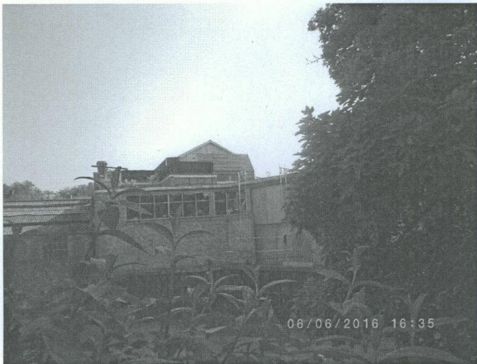
South elevation from Haggerston Bridge
